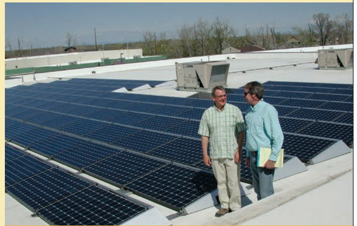
Robert Gibson (l.) and Mark Shyne (r.) stand near SIMMS solar electric array, the fifth largest in the state.
